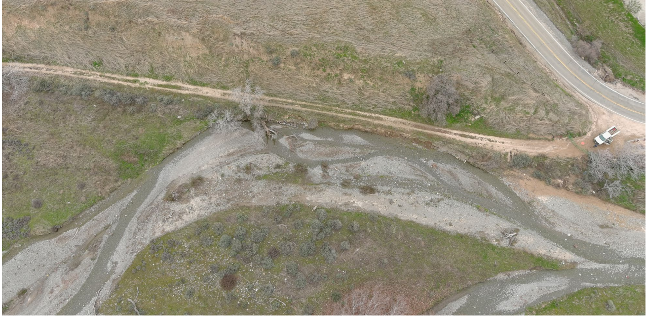
Figure 2-27: Drone photo of the emergency repair at the Tesla property.
