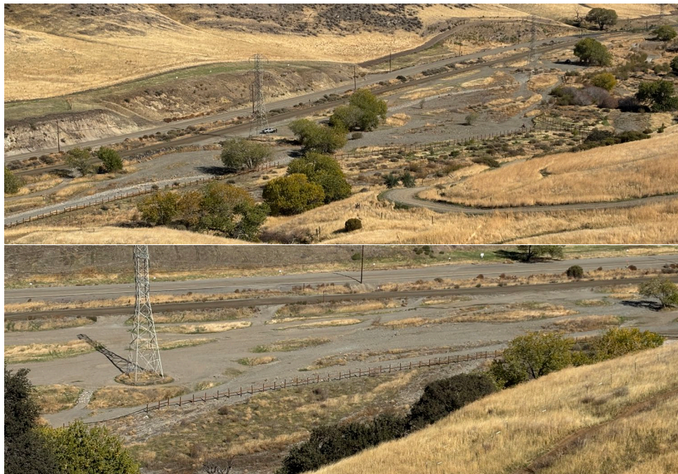
Figure 2-24: Completed creek delineation fencing at Corral Hollow Creek.
